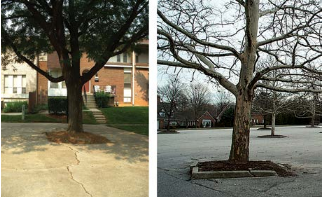
Figure 39. Trees planted in holes that are too small may eventually crack nearby pavement.
