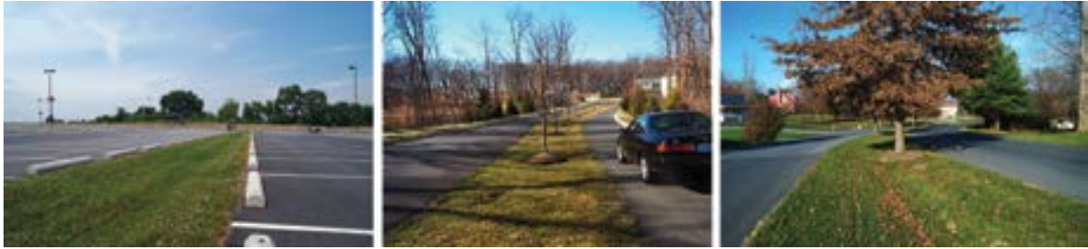
Figure 18. Swales with trees offer greater benefits than a swale with no trees (left).
