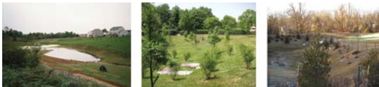
Figure 17. Storm water ponds with trees incorporated offer benefits over a conventional storm water pond with no trees (left).
