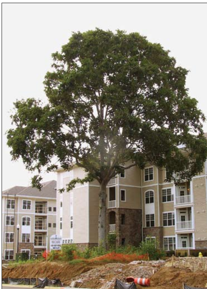
Figure 17. Specimen tree protected during construction.
