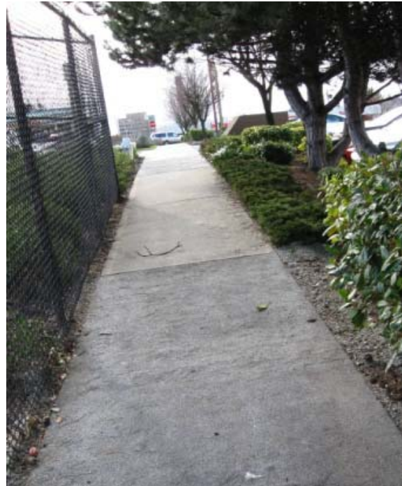
Installation of alternative sidewalk material
