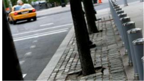
A continuous trench with pavers
