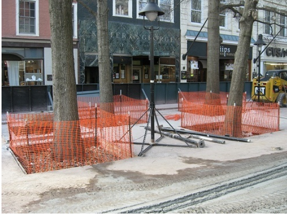
Fencing used around trees to help protect them through construction.
